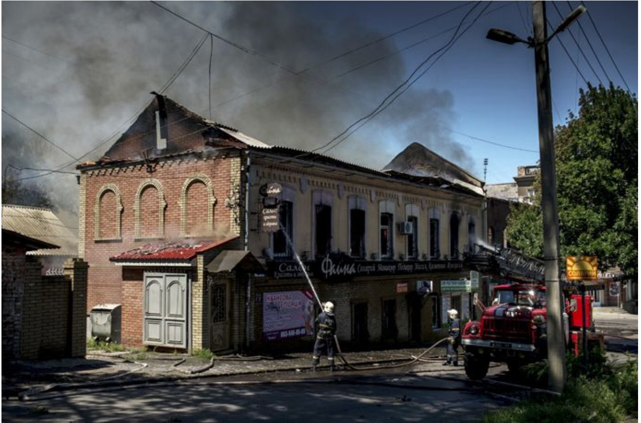
Fire brigade members extinguishing fire in a building hit by a shell during an artillery attack by the Ukrainian Security Forces in Lugansk. (RIA Novosti/Valeriy Melnikov)
